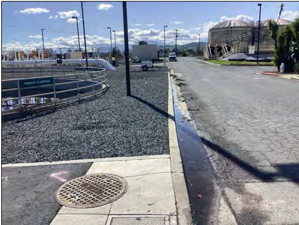
Photo 2. Area of planned pipeline in project area within WWTP (looking south).
