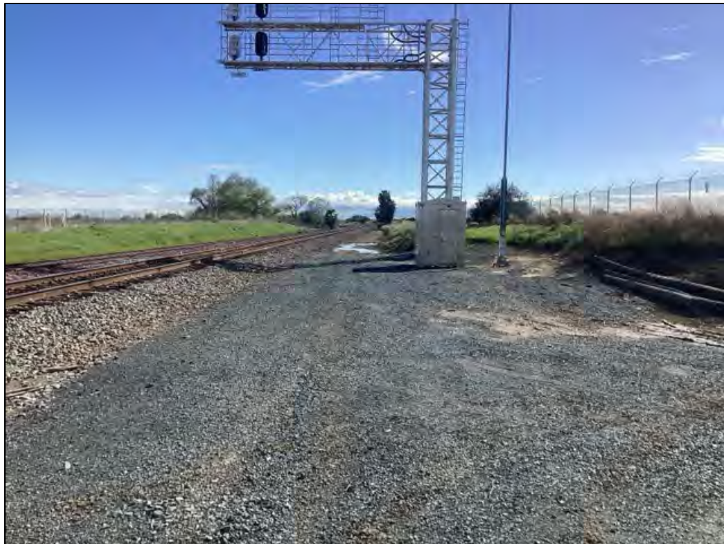
Photo 15. BNSF railroad tracks north of project area and WWTP (looking east).
