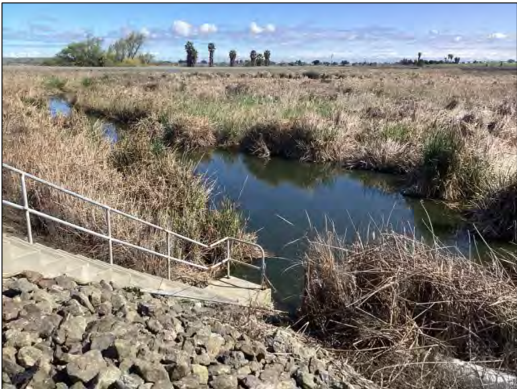
Photo 12. Emergency retention basin north of project area within WWTP (looking northeast).
