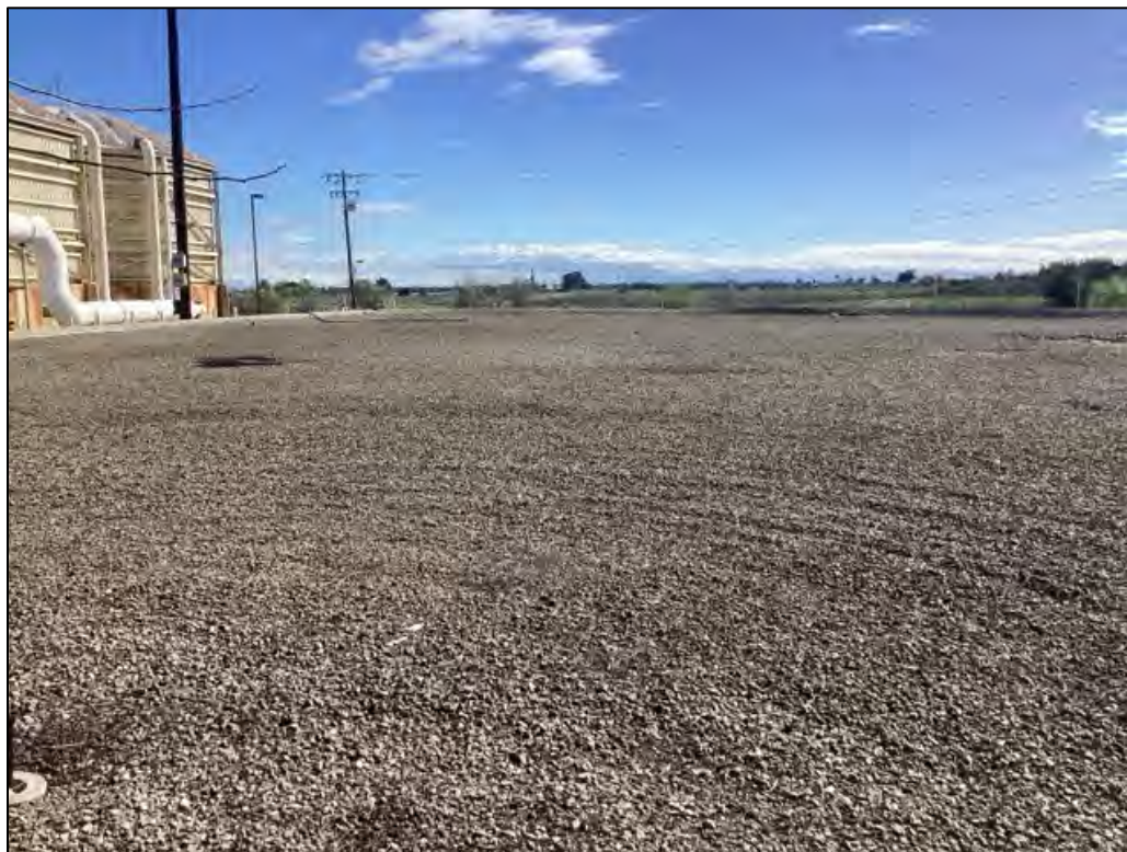
Photo 5. Area south of trickling tower filters and odor control biofilter facility in project area within WWTP (looking east).
