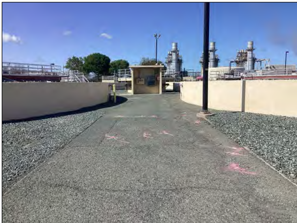
Photo 6. Area of planned pump station in project area within WWTP (looking east).
