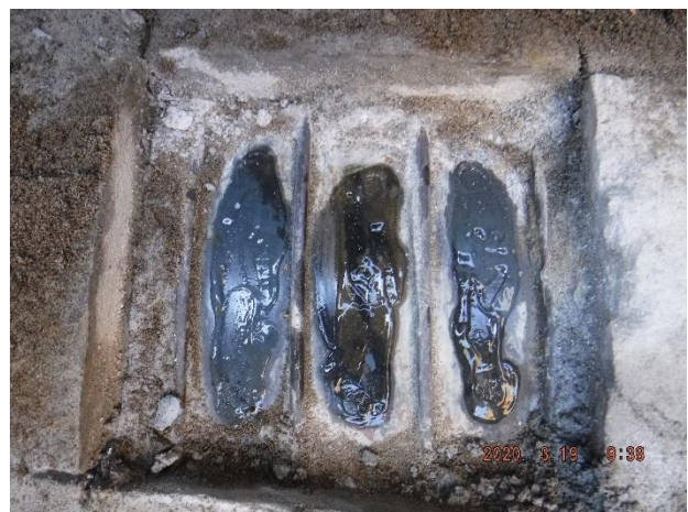
Photo 4-10. Exposed steel area at Location 4. Surface is wet from ultrasonic testing.
