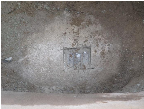
Photo 4-7. Exposed pipe surface at Location 2.
