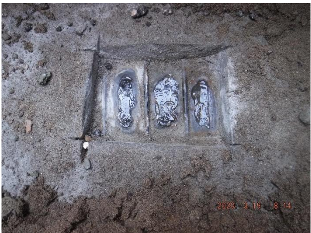
Photo 4-15. Exposed pipe surface at Location 7.
