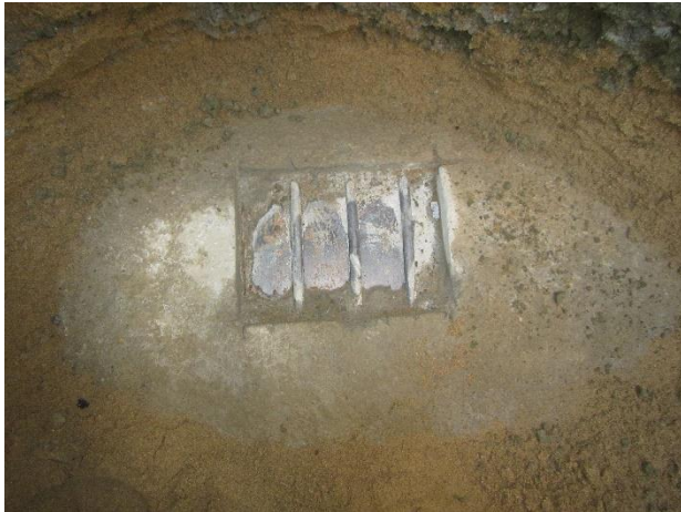
Photo 4-3. Exposed pipe surface at Location 9.
