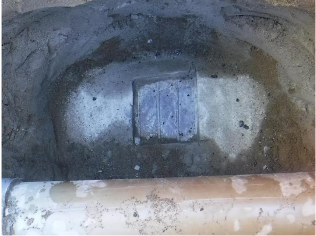
Photo 4-11. Exposed pipe surface at Location 5.
