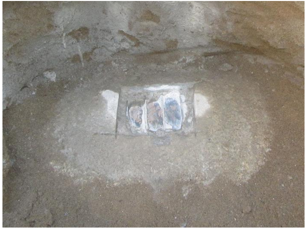
Photo 4-17. Exposed pipe surface at Location 13.
