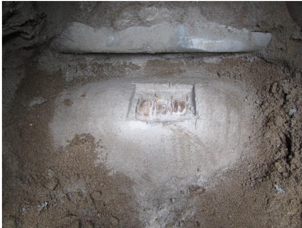
Photo 4-5. Exposed pipe surface at Location 1.
