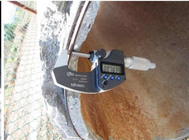
Photo 4-2. Sections of pipe removed from AFM102 have a cylinder thickness of approximately 14 gauge (0.075 inches). The measured thickness was 0.078 inches, possibly including the rust.
