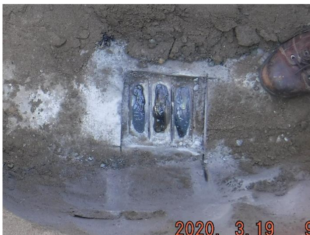
Photo 4-9. Exposed pipe surface at Location 4.
