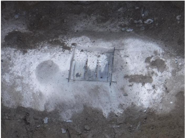
Photo 4-13. Exposed pipe surface at Location 6.
