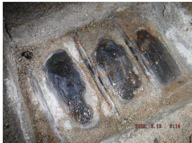
Photo 4-16. Exposed steel area at Location 7. Surface is wet from ultrasonic testing.
