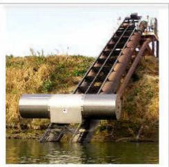
A track allows the screen to be pulled up for inspection or non-use periods.
